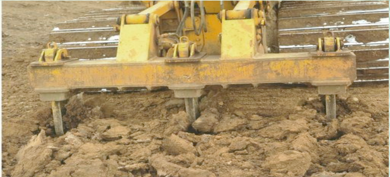
Ripping Compact Subsoil
