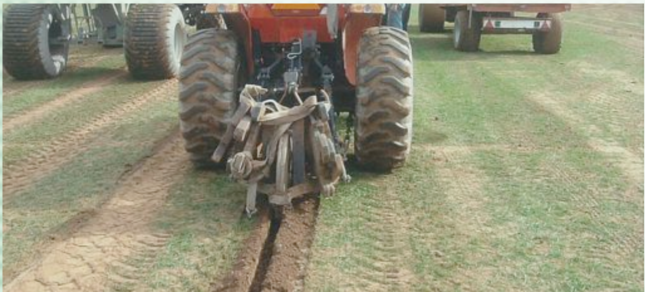
Packing the Gravel fill of the Slit
