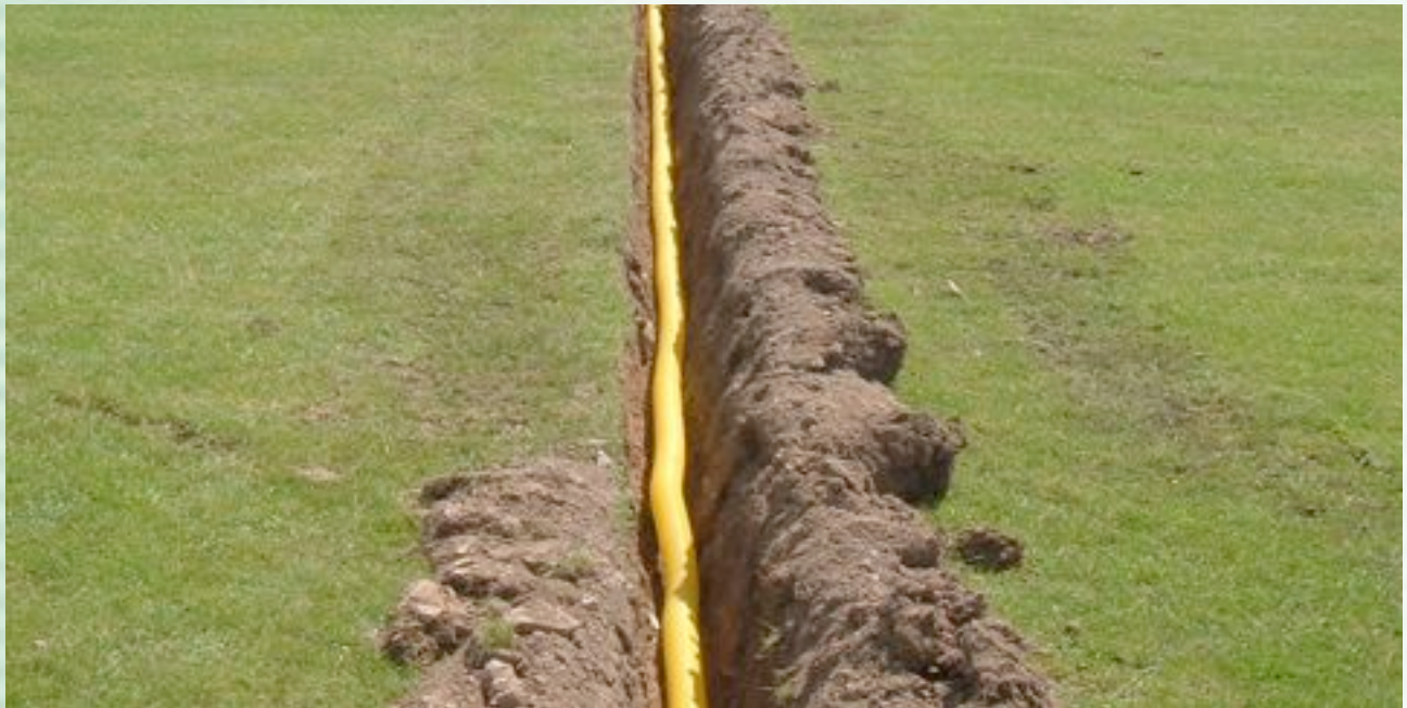
Drainage pipe laid in Lateral
