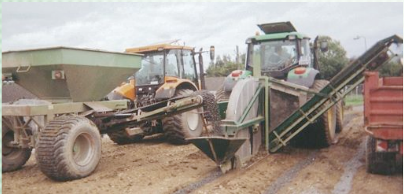
Slit Drainage in New Pitch Construction
