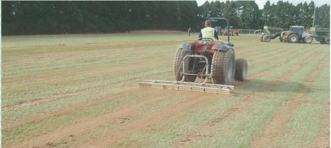
Brushing and Levelling the Sand in the slits
