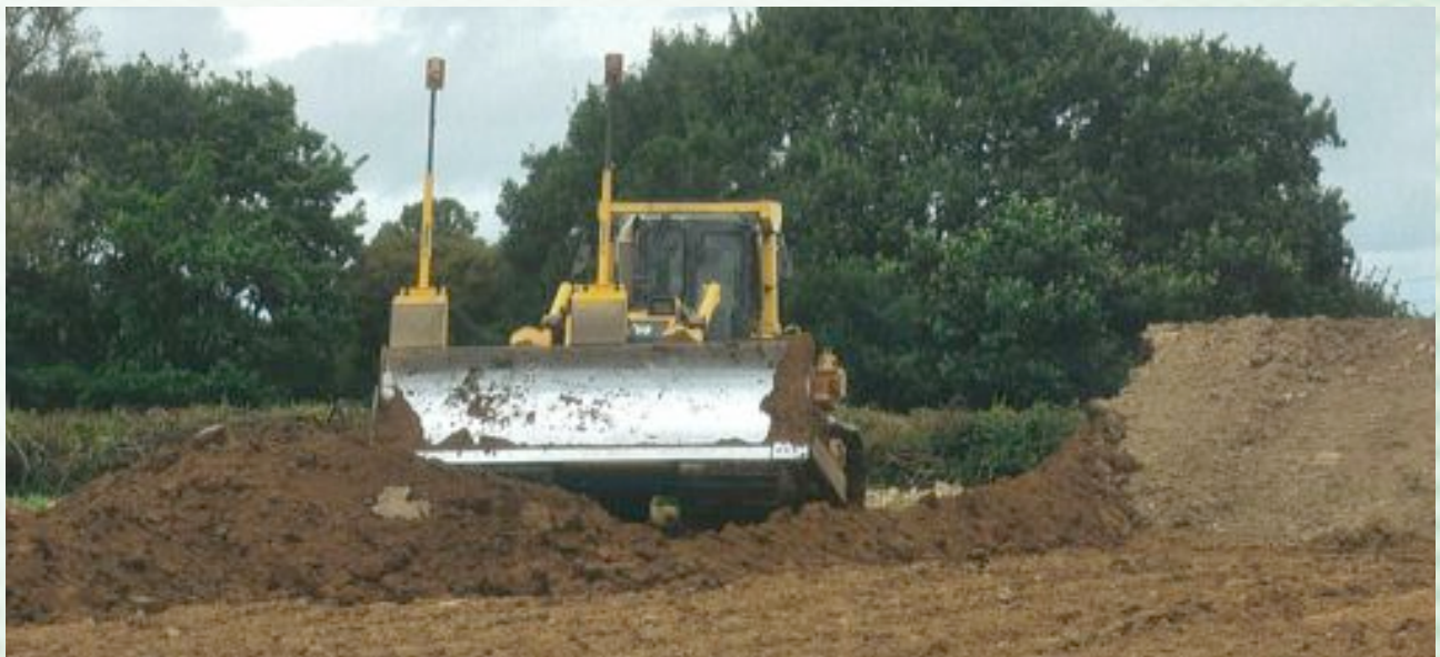
Pushing Back the Topsoil with Lazer Controlled Dozer.
