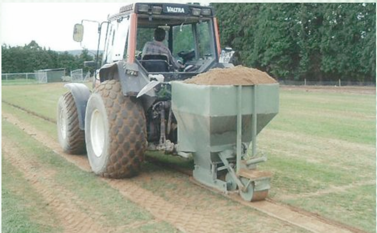
Slit Drain bein Topped with sand
