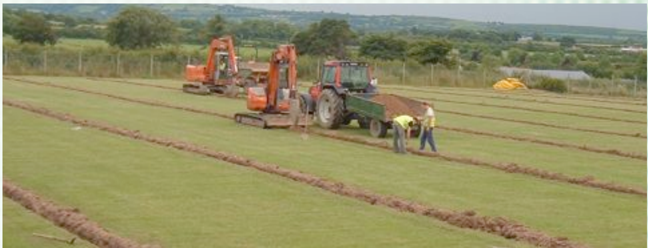
Pitch with a number a Lateral Drains in place
