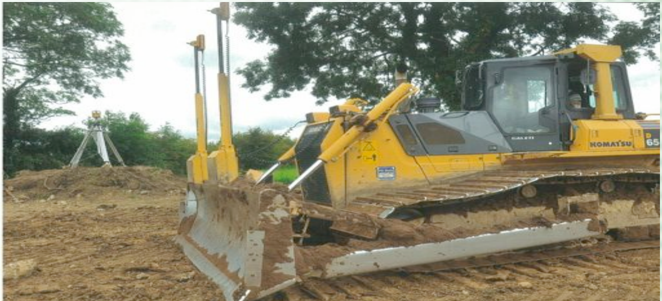
Laser Station and Dual receivers on Dozer
