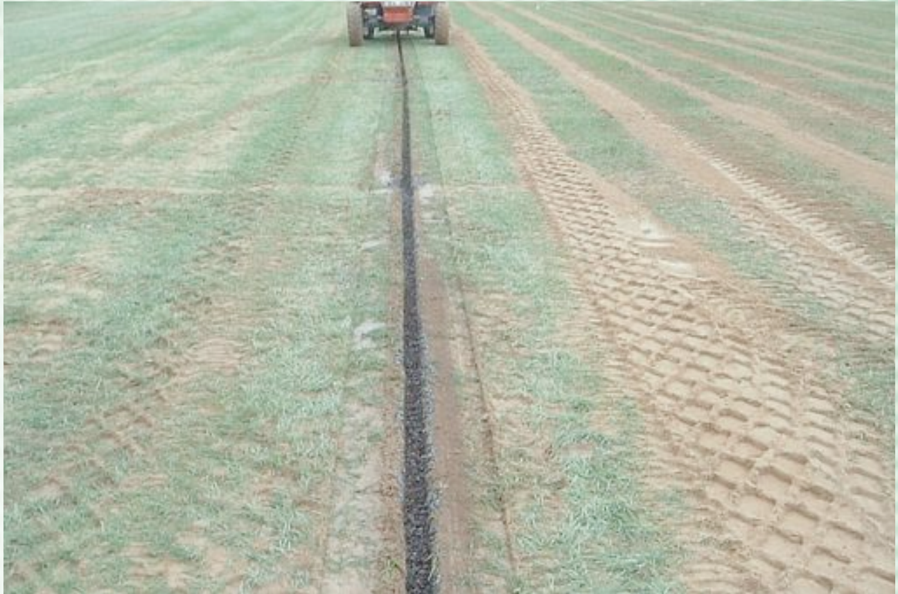
A Slit Drain with Gravel Fill
