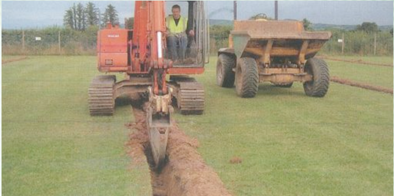
Excavating a Lateral Drain
